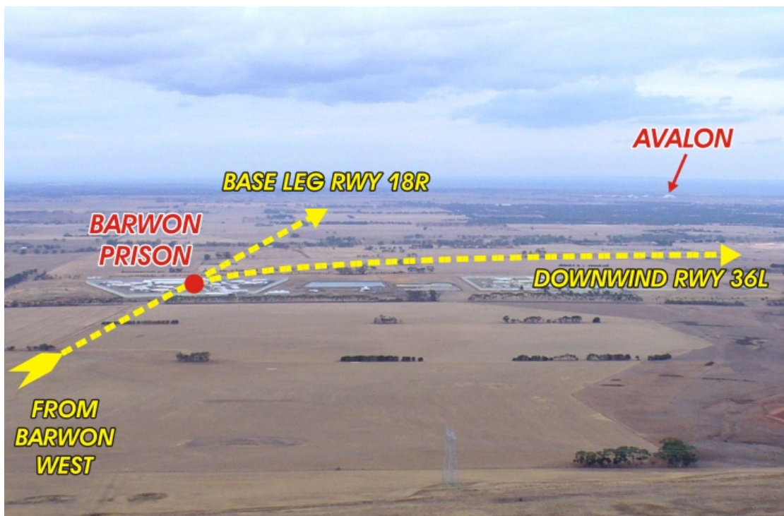
Above: Approaching BARWON PRISON, looking east.
